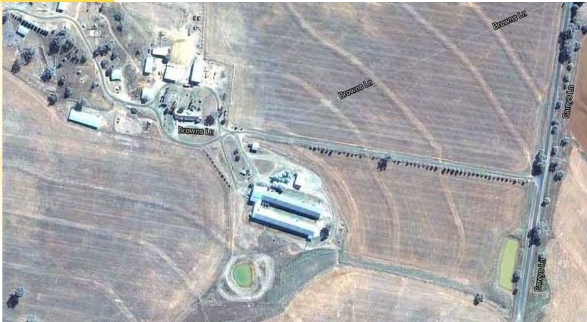
Figure 5-1: Aerial view of Glendon farm Tamworth. A-Cage system for older birds; B-barn type system for younger birds 0-15 weeks
